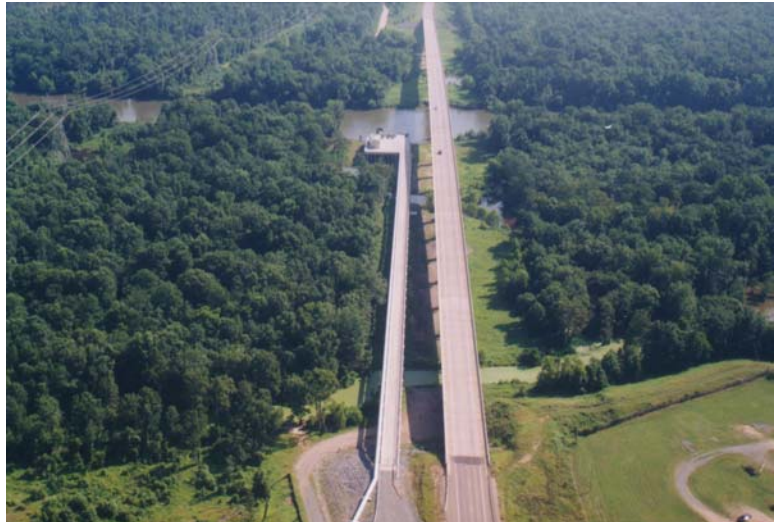
Phase I: 65 mgd Charles E. Thomas intake west of Ouachita River Bridge/Highway 167 (facing north)
