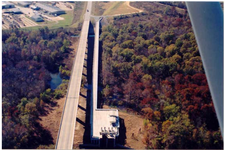
Phase I: Intake west of Ouachita River Bridge/Highway 167 N (facing south).
