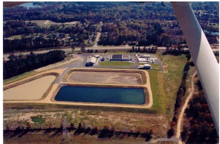
Phase I: Sherrel F. Johnson Clarification Facility (facing
